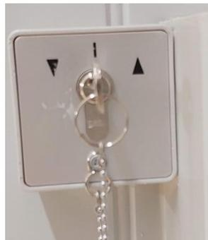
To manually lower or open the shutters, turn the key toward the up or down arrow as needed and hold in that position until the shutter has reached the desired position.
